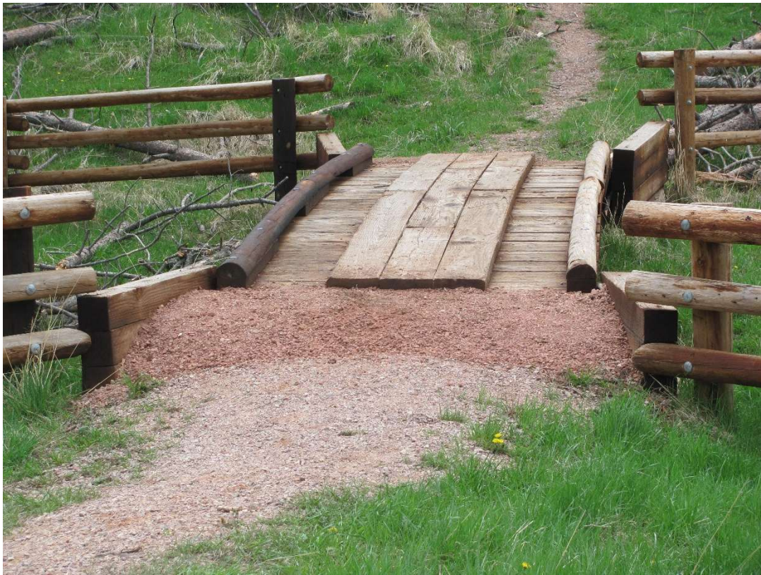
Figure 16. Palmer Creek bridge on Trail 2 in 2013. BH BCH spread gravel on bridge approaches in May 2013.
