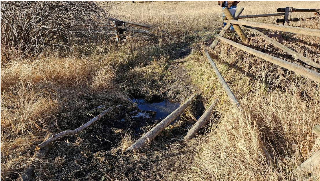
Figure 17. Palmer Creek crossing at old bridge site on Trail 2 in Spring 2025.
