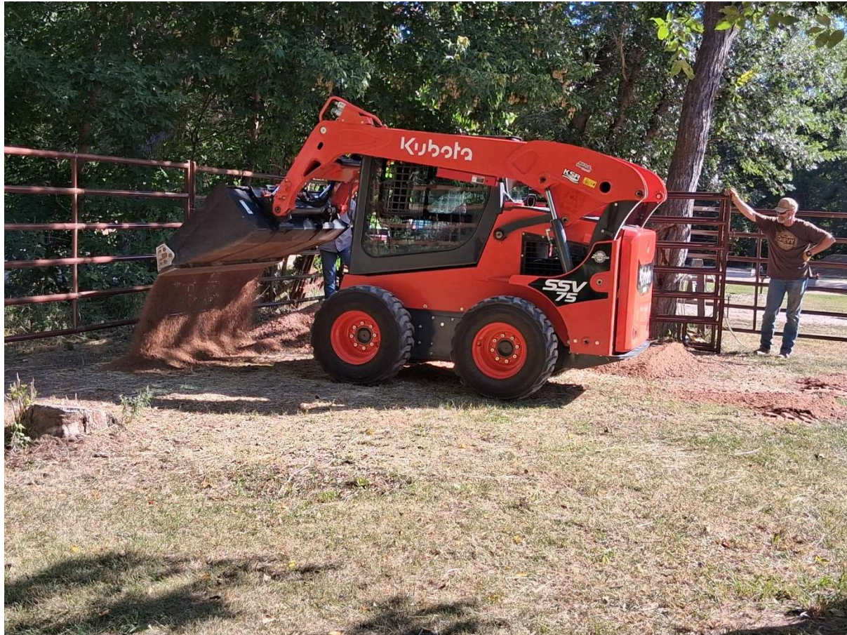
Figure 13. Doug with his skidsteer placing gravel inside the new corrals.
