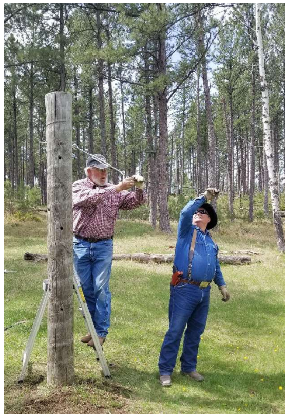
Figure 10. Doug and Jim tightening the highline.
