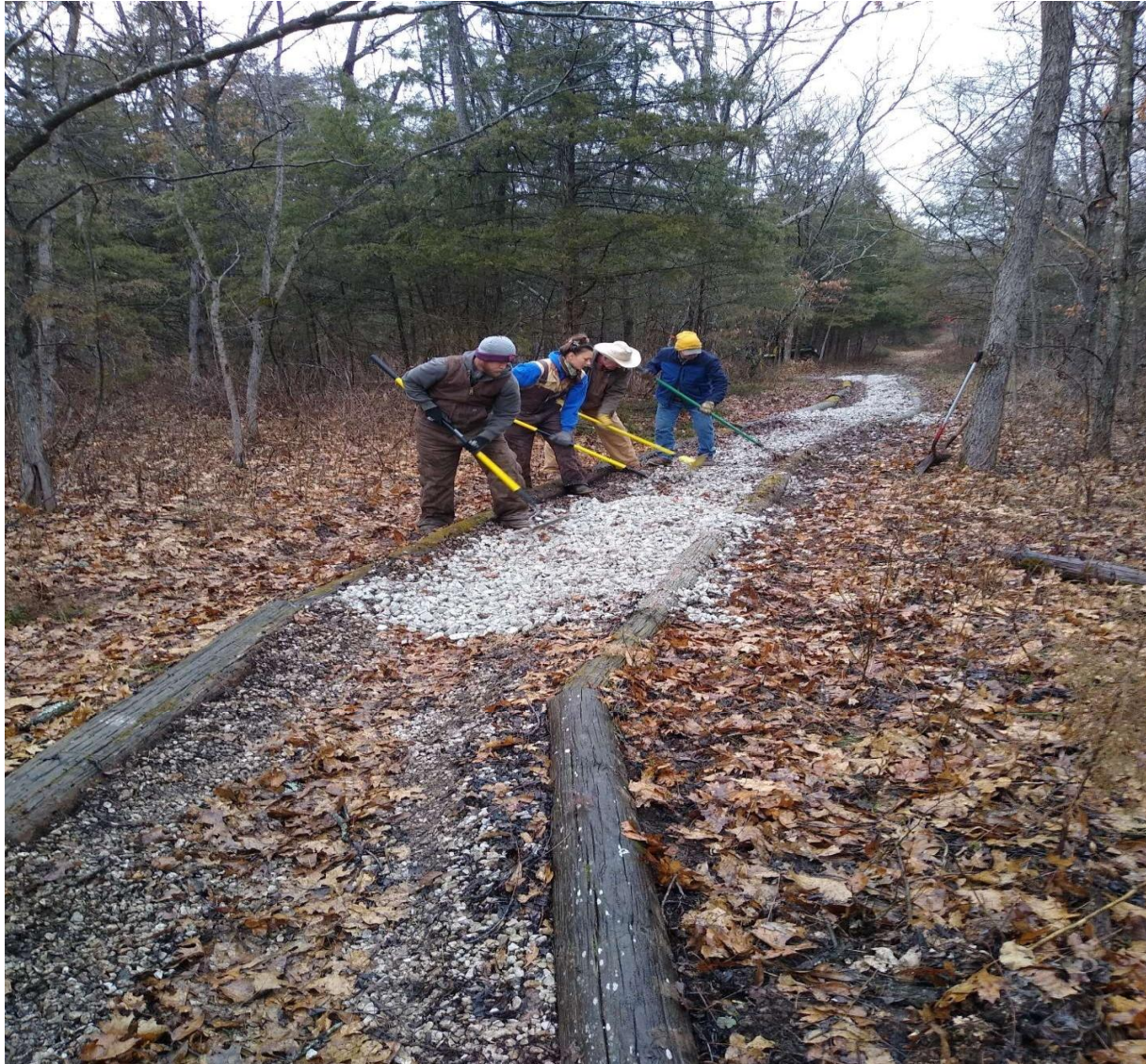
Placing gravel along the tread of the trail.
