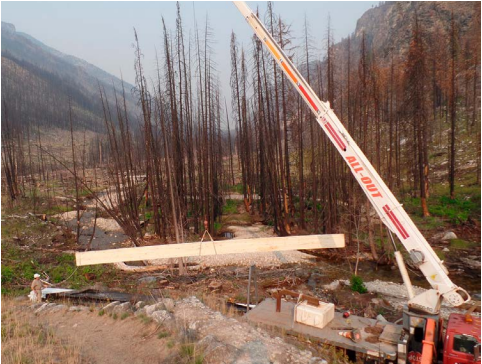
Photos from top: Abutment beams hauled to creek sides using old-fashioned muscle power! Crane swings laminated beams into position. MCC and FS crew members prove that moving rocks ROCKS! SPWBCH volunteers proud of the new bridge over Roaring Lion Creek.
